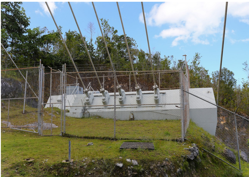
Figure 2: Tower anchor, showing the seven cables.
